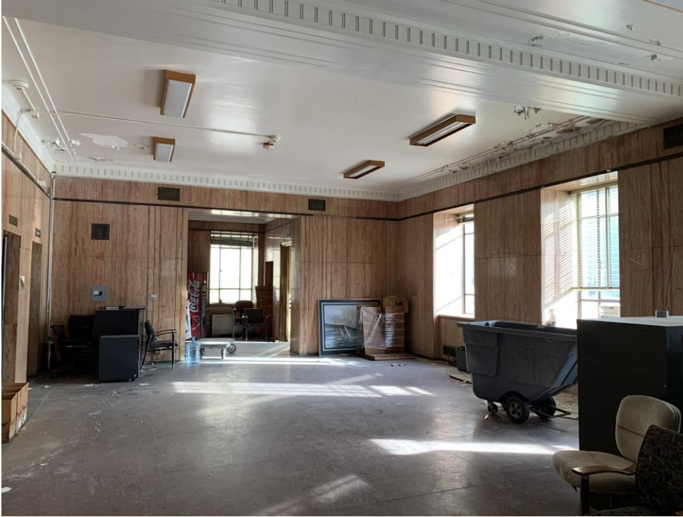
Interior view looking west from middle of lobby 13 of 23
