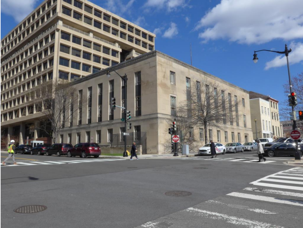
General view looking northeast showing south and west elevations 1 of 23
