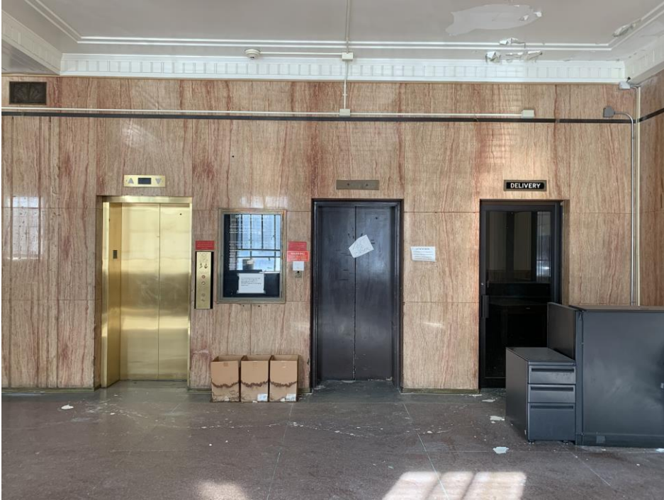
Interior view looking from lobby to elevator bank on north lobby wall 15 of 23
