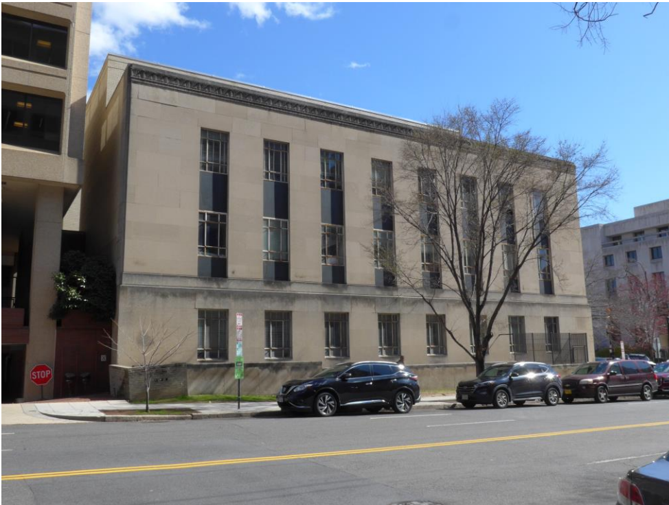
View looking southeasterly showing west elevation 2 of 23
