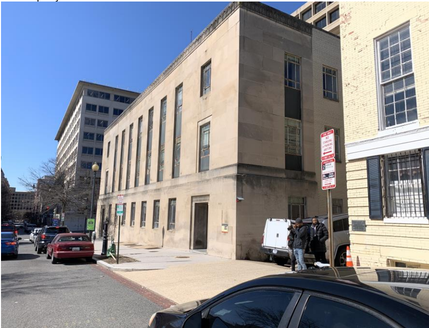
View looking west showing south and (part of ) east elevations 5 of 23
