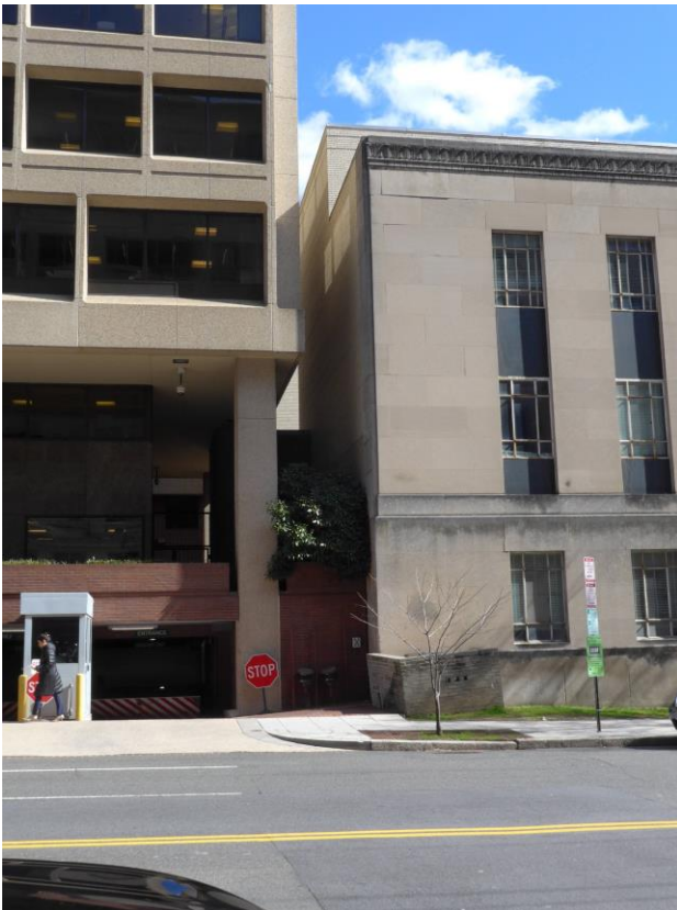
View looking east showing north elevation of building abutting passageway between the Recorder of Deeds and adjacent building to the north 4 of 23
