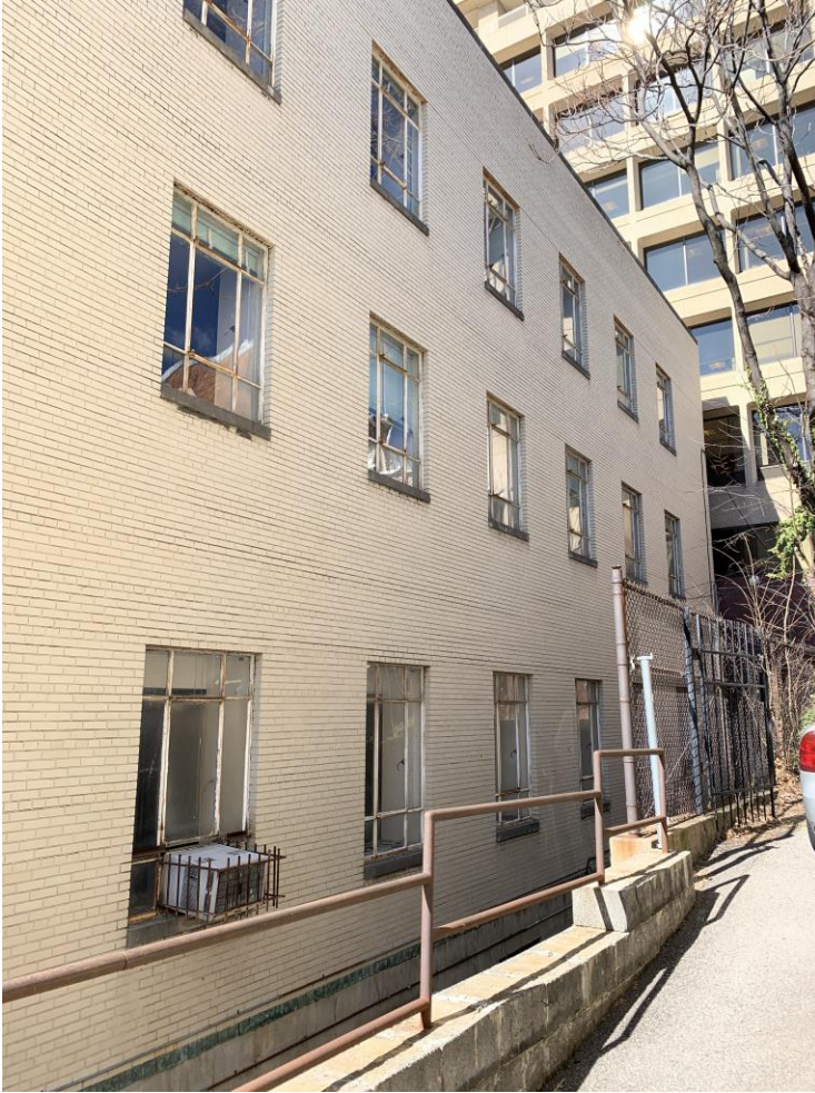
View looking north showing east elevation 8 of 23
