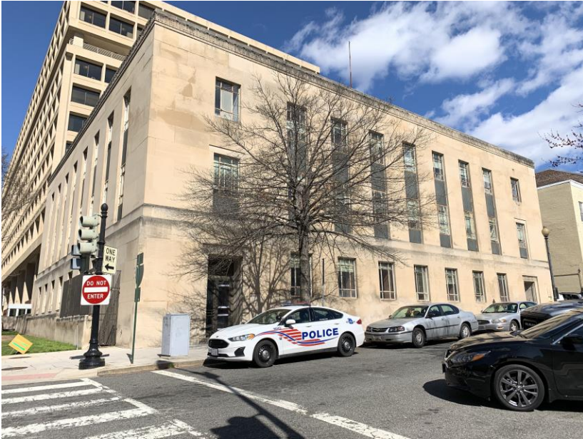
View looking northeast from corner of 6 th and D streets 3 of 23
